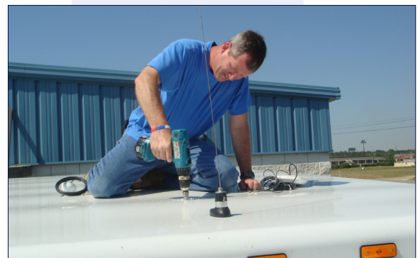
Doug Brownlee of Macon Communications installs the AVLS in a Laurens County EMS ambulance during the pilot vehicle installation on April 23, 2010.
